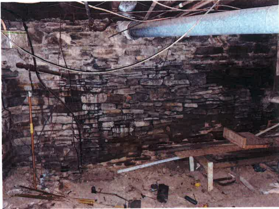
Basement looking South
