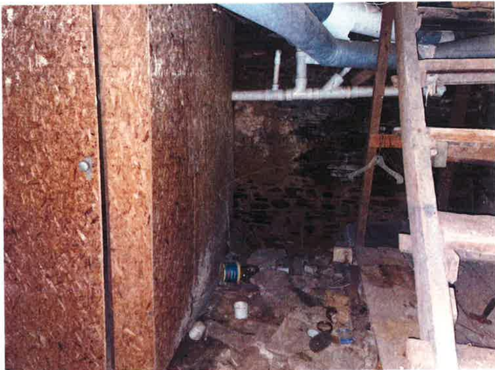
Basement looking North
